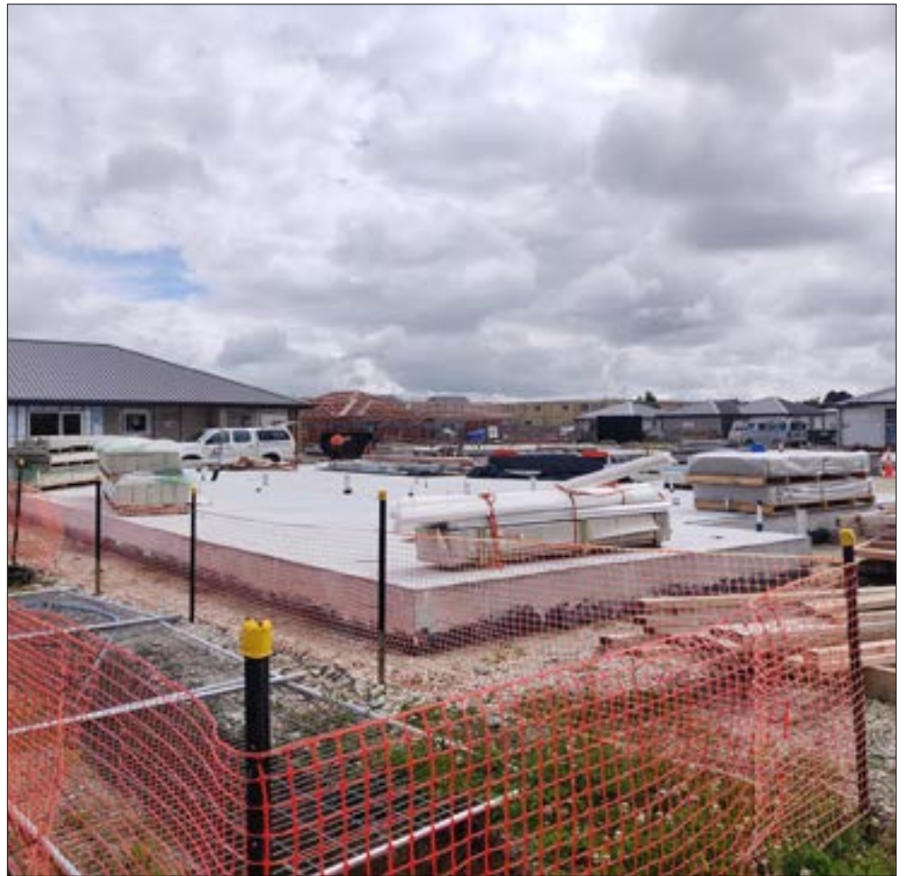
The village under construction
